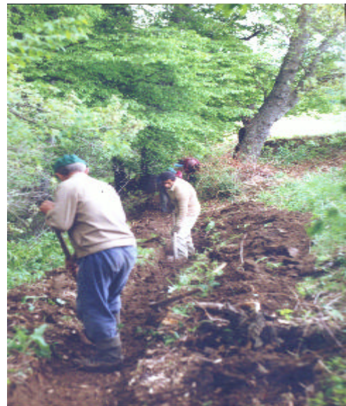
Workers building a water supply channel
