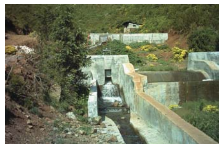
Republic of Albania Mountain Areas Development Programme Captation of spring water constructed with the support of IFAD. Water is used for around 300 families and 180-200 ha. A basin is present in the upper part where trout are bred.
