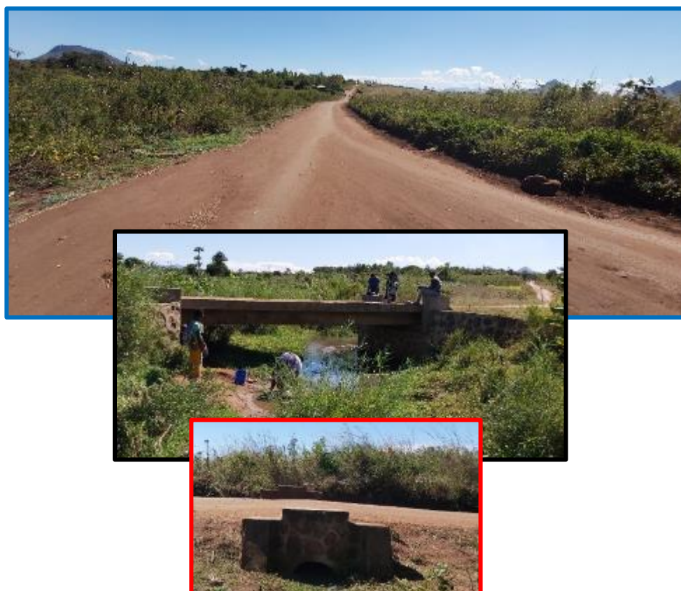
Figure 5-6 RLEP Rehabilitated Roads in Thyolo
