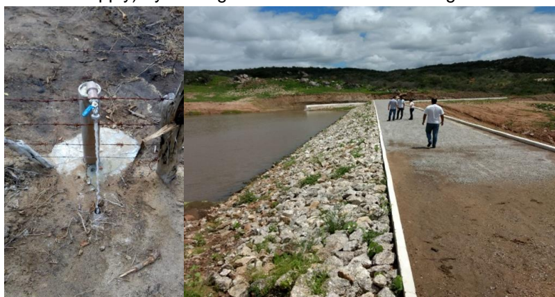
Picture - Water security strategies supported by PROCASE. Right: large dam to collect surface water ( Riacho Fundo , municipality of Tenório ). Left: Deep Tubular Well implemented in benefited community. Source: PROCASE, 2019.
