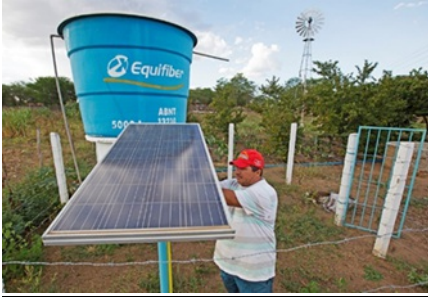
Picture 5 - Emergency Plan - Irrigated fields: Installing the water well, water tank and solar panel of the irrigation kit. Source: Semear International Programme.
