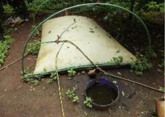
As microbes digest the organic material, biogas bubbles up from the mixture, inflating the plastic bag. Sitting above the ground in the sun, the system quickly heats up, promoting rapid production of methane gas. It is then piped through a PVC tube connected to an appliance or piece of equipment such as a gas stove for cooking.
