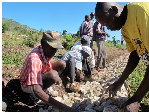
Haiti - Small-scale Irrigation Development Project, Calon Nan Jules, North-west region. Men build stone barrages on the upper watershed slopes
