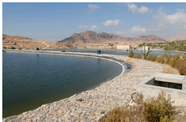
Jordan - Agricultural Resource Management Project - Phase II. Polishing ponds are used to expose water to the sun for one month to remove bacteria.
