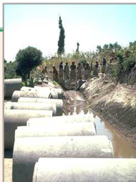
Cement tubes dug vertically in the basin bottom to realize a siphon-like system.
