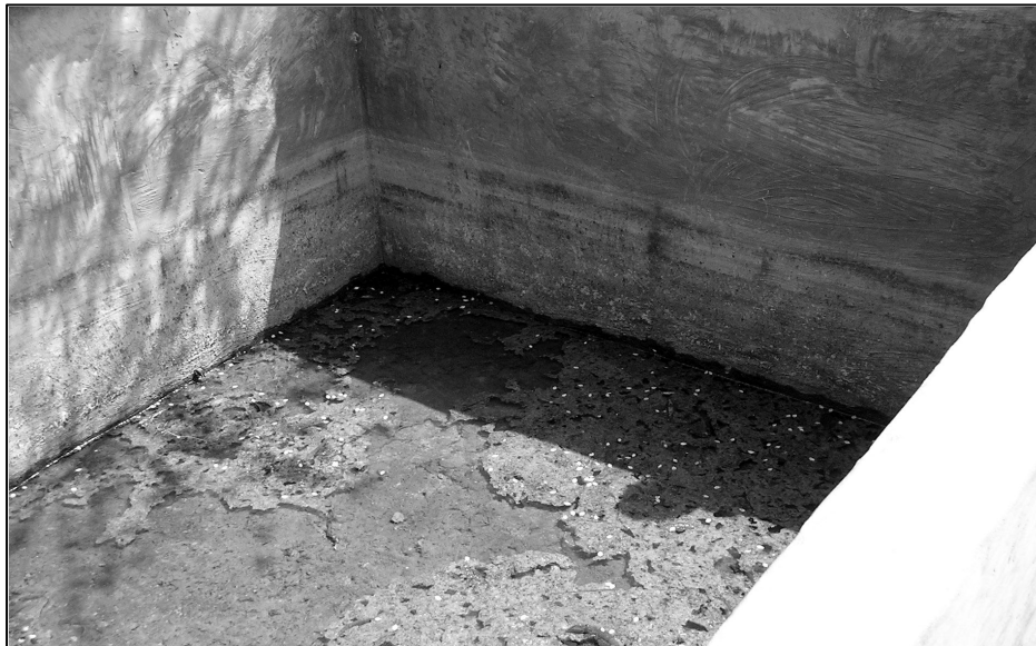
A rainwater storage tank that clearly never even got half full. There were serious weaknesses in the design, construction quality, capacity for storage and water quality assurance of storage tanks. IFAD photo by Michel van der Stricht
