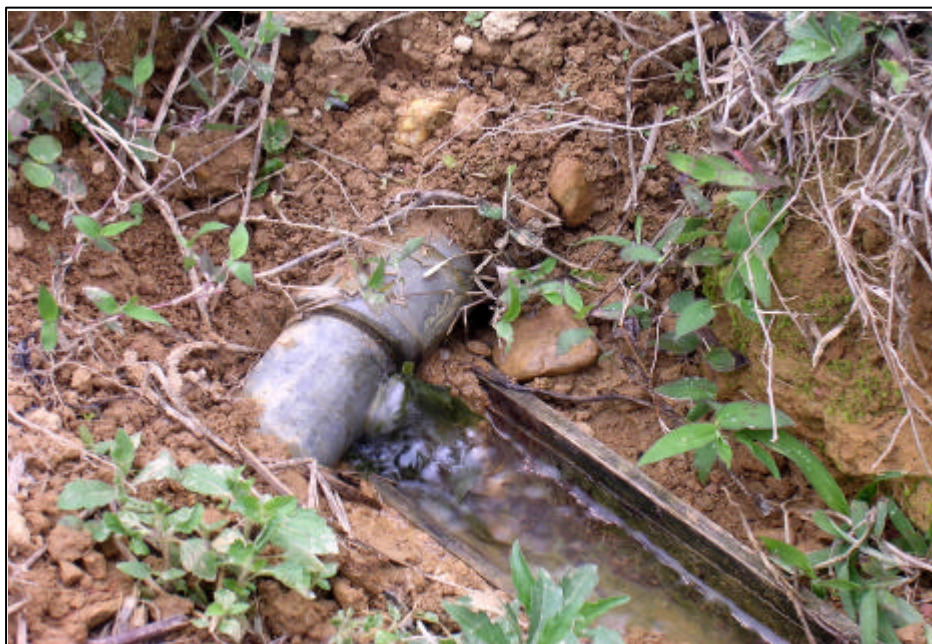
A gravity flow system (to collect water running off the hills) in Ngog Long, Yen Minh. Here, the supply pipe leading to the drinking water tank has been illegally diverted to irrigate private land – fairly common practice. With better supervision such piracy could have been better monitored and minimized.
