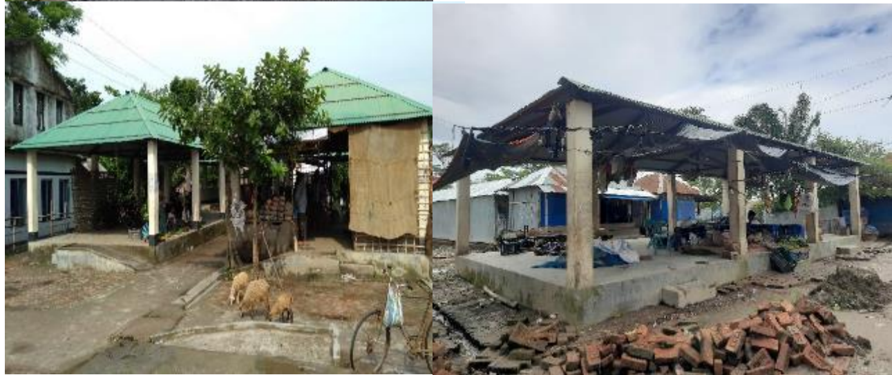
Munshiganj Bazar, Shyamnagar, Satkhira
