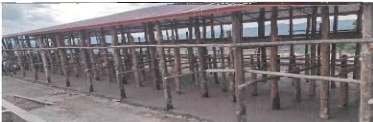
The construction of Rwaniro/Huye Communal cowshed, Huye District, May 2021
