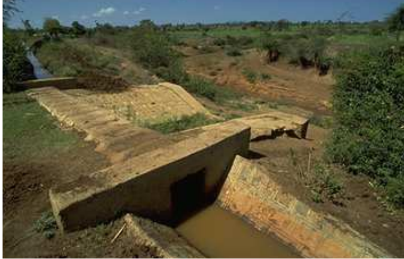
A dam on the Nego river which forms part of the irrigation system built by an IFAD project (Rehabilitation Programme for Drought Affected Areas). Note the gabions, stones lining the river bank and being kept together by a metallic net. This irrigation scheme will benefit farmers of cooperatives in the area.
