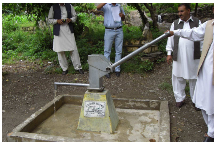
Water pump for accessing drinking water.
